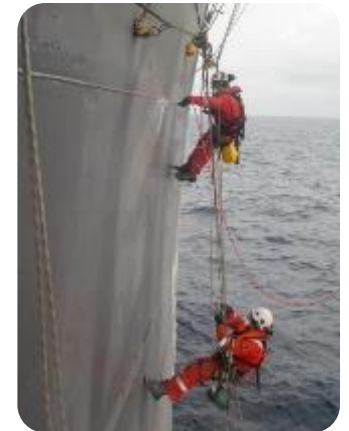
Painting and Blasting Services
