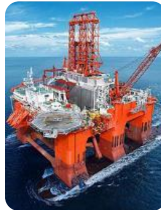
Inspection of Offshore Installations: FPSO, MODU, Fixed Platforms
