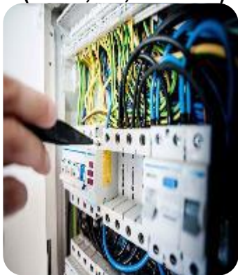
Inspection of Electrical Installations (ATEX, CP, DCVG...)
