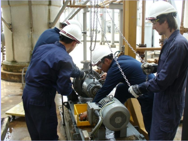
Pump Removal / Replacement
