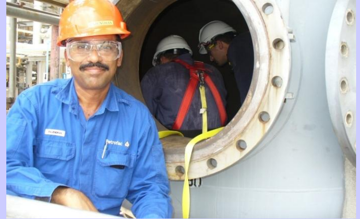
Vessel Entry & Inspection
