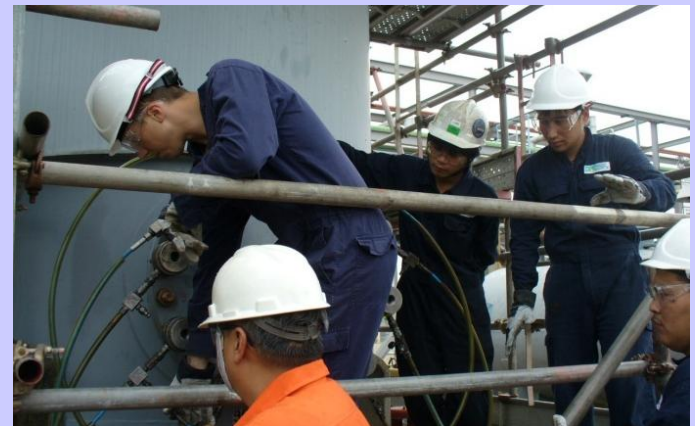
Bolt Tensioning
